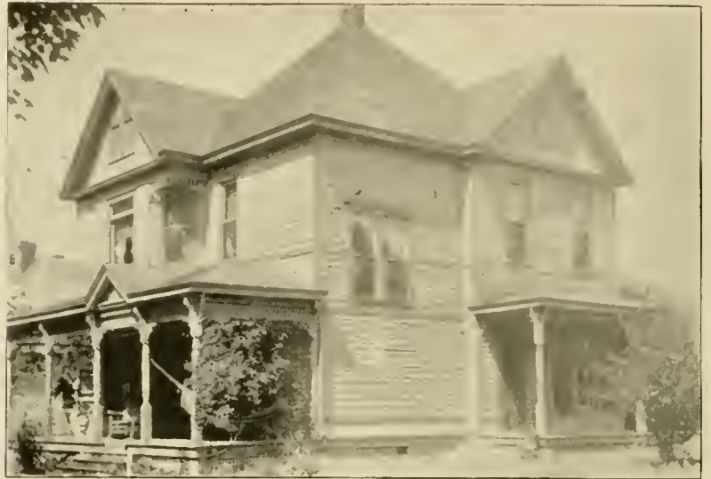
RESIDENCE OF T. N. LAKIN. North 1st Street.
